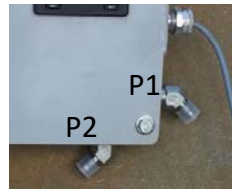
Control valve connections on control panel.
