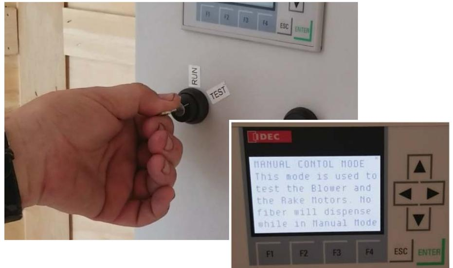
While one person watches the end of the rake motor housing (through the fan guard), the other person momentarily presses the **RAKE** button on the control panel. As the motor slows to a stop, the direction of fan rotation should be evident. Confirm that the fan is rotating counterclockwise, as indicated by the arrow on the end of the motor housing.
