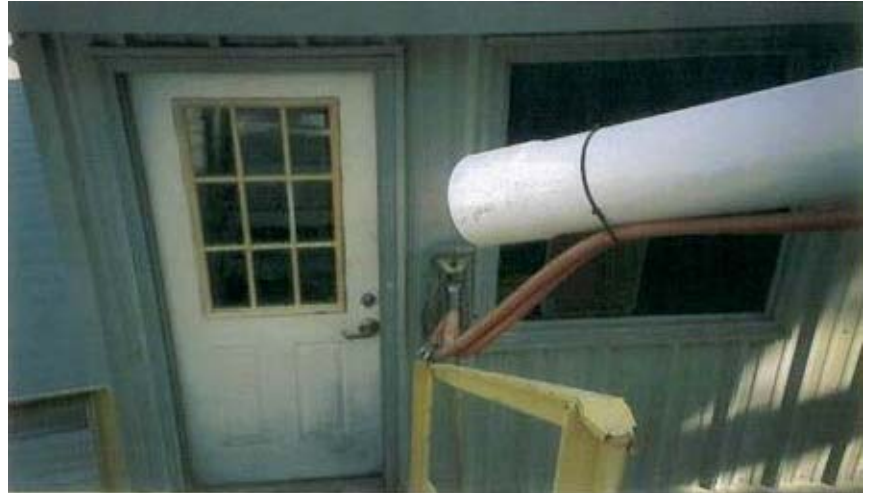
Fiber addition point located near product storage area.
